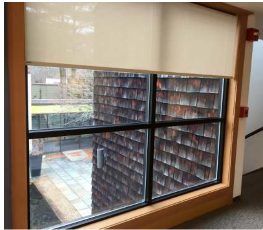
Installation of New Insulated Windows
