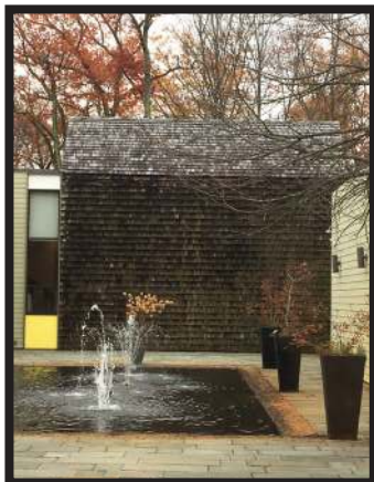
Repair of the Sloped Rooftop Shingles
